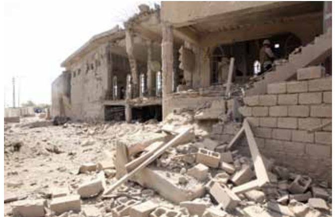
Camp Ramadi, Iraq, April 22, 2008. Destruction caused by the blast of a large quantity of explosives a suicide bomber detonated after attempting to get through an entry control point. Recognizing the threat, LCpl Jordan Haerter and Cpl Jonathon Yale engaged the truck with precise fire. The two Marines were mortally wounded. Their actions saved the lives of 50 Marines and Iraqi policemen. 2ndmardiv.marines.mil
